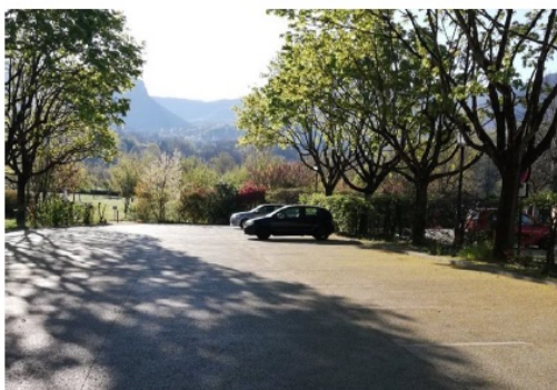
Parking en béton poreux, Beauvoir-en-Royans (illustration)
